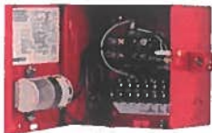
Capacitor in Standard Control Box 410861-001
